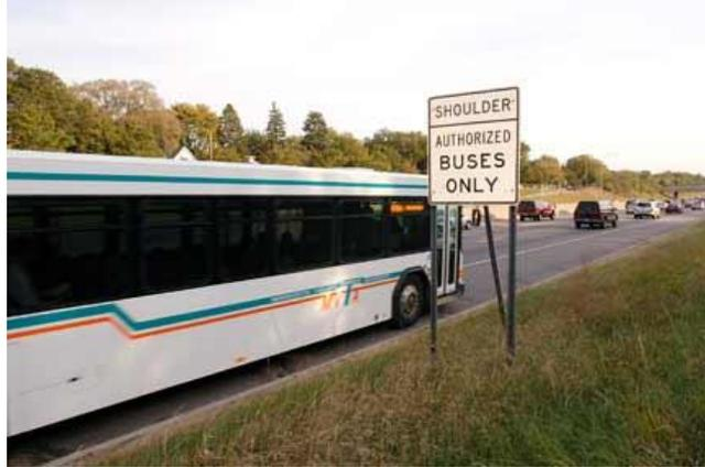
*Figure 1: An example of a bus bypass shoulder. Source: MnDOT*
