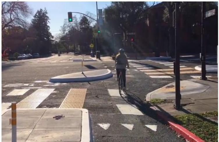
*Figure 3: Protected intersection installed in Berkeley. Source: Susie Hufstader, Bike East Bay*
